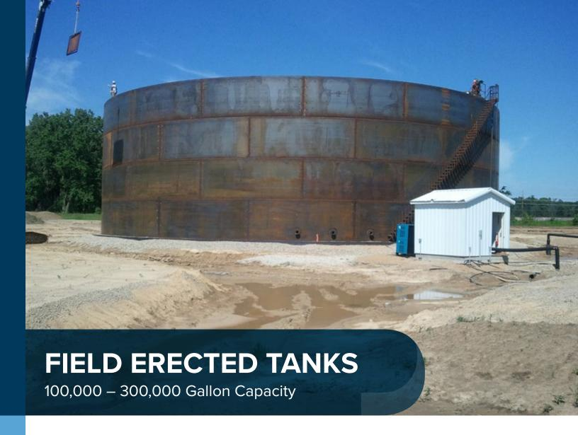
Precision Tank specializes in welded above ground steel tanks used for storage of liquid fertilizer, fuel, water, chemicals and other bulk commodities.
